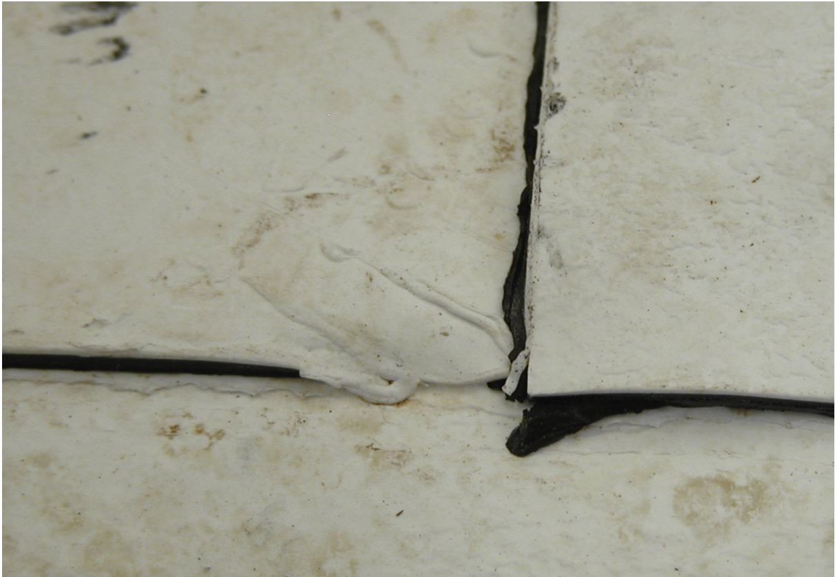
Figure 3: Sheet surface with T joint
